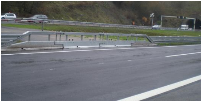
Protection of an emergency opening, single-lane
