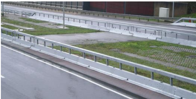
Protection of an emergency opening, dual-lane
