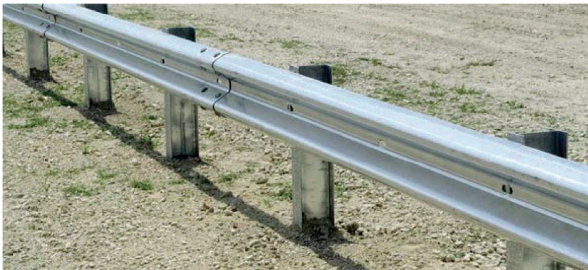
Figure 1 : Traditional steel guardrail
