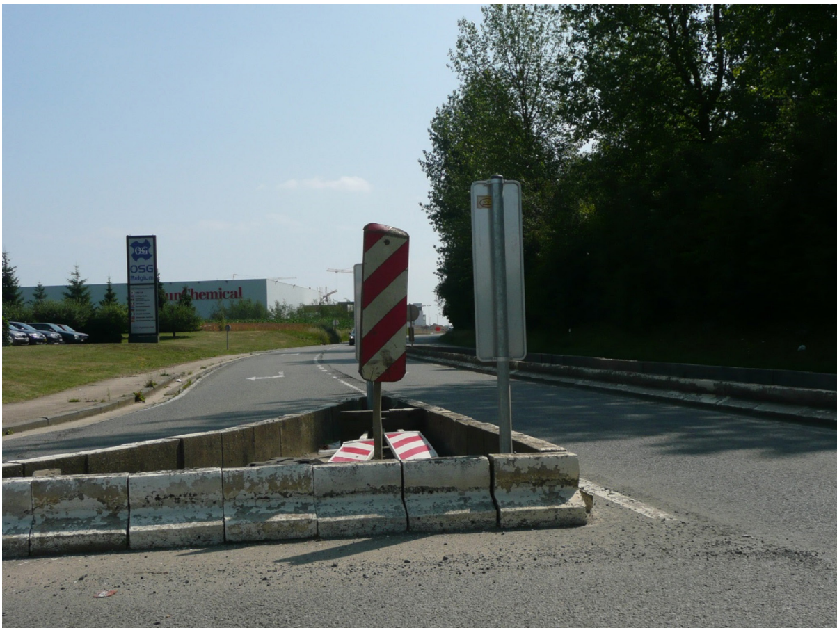
Figure 8 : Obstacles blocking the view at a cross road
