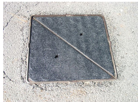
Figure 11 : Manhole cover after anti-skid treatment
