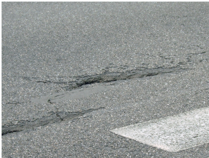
Picture 6: Potholes/fissures
