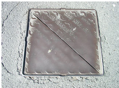
Figure 10 : Manhole cover before anti-skid treatment
