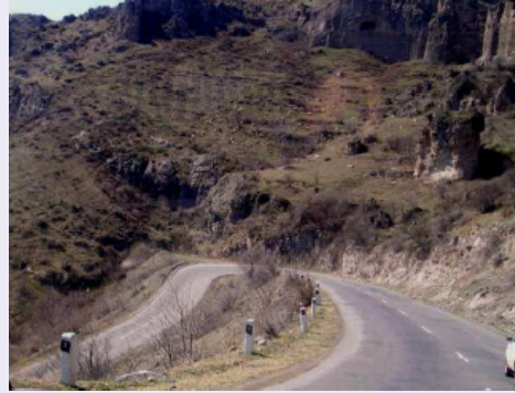
Steep embankments represent a severe roadside hazard for car occupants involved in a run-off road crash (risk factor = 5.00)
