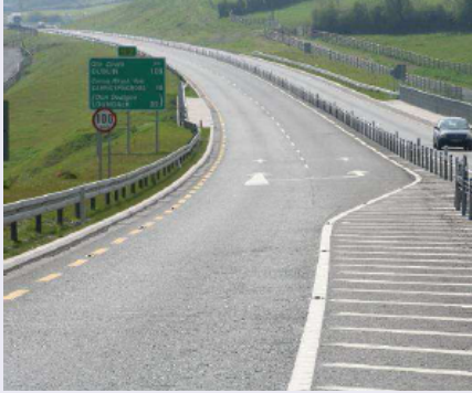
Safety barriers help reduce the kinetic energy of a run-off road crash for car occupants (risk factor = 1.75)
