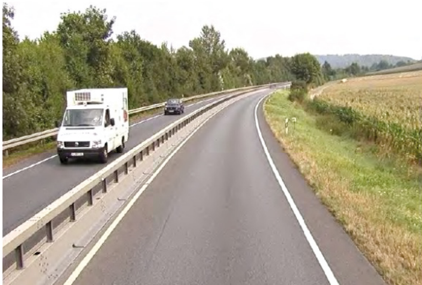
Situation after Installation
