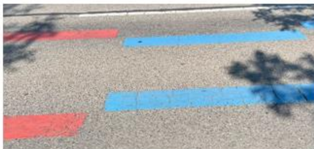
Picture 3 Old road markings at Siemensstraße in Vienna/Austria exposed to an average daily traffic 16000 vehicles
